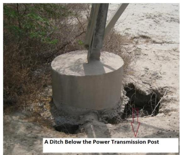
**Fig. 4.** Development of a ditch.
