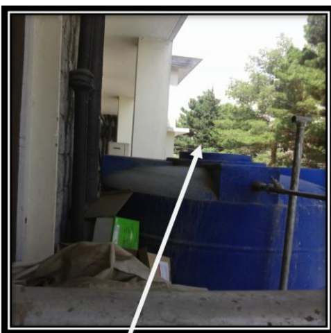
Fig. 4. Overhead tank without cover at DHQ Hospital.
