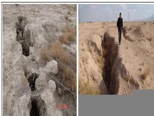
**Fig. 5.** Tension cracks due to land subsidence in Tous area.
