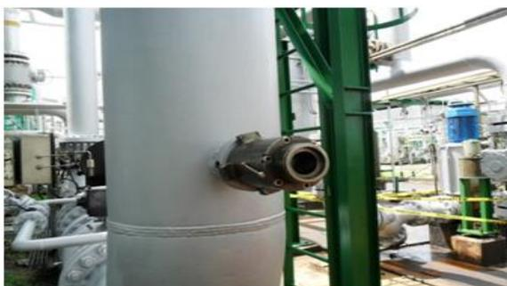
**Fig. 2.** Access valve of oil pipeline for insertion of coupons.
