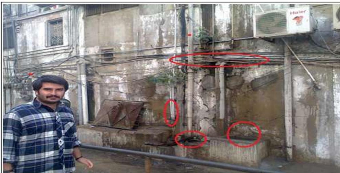
**Fig. 7.** Shows drinking water pipes association with sewage line (Block 6).
