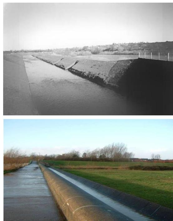
**Fig. 2.** Side weirs in channel.
